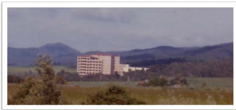
Vista general del hospital
