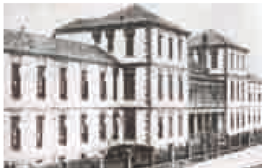
HOSPITAL SAN ANTONIO ABAD
